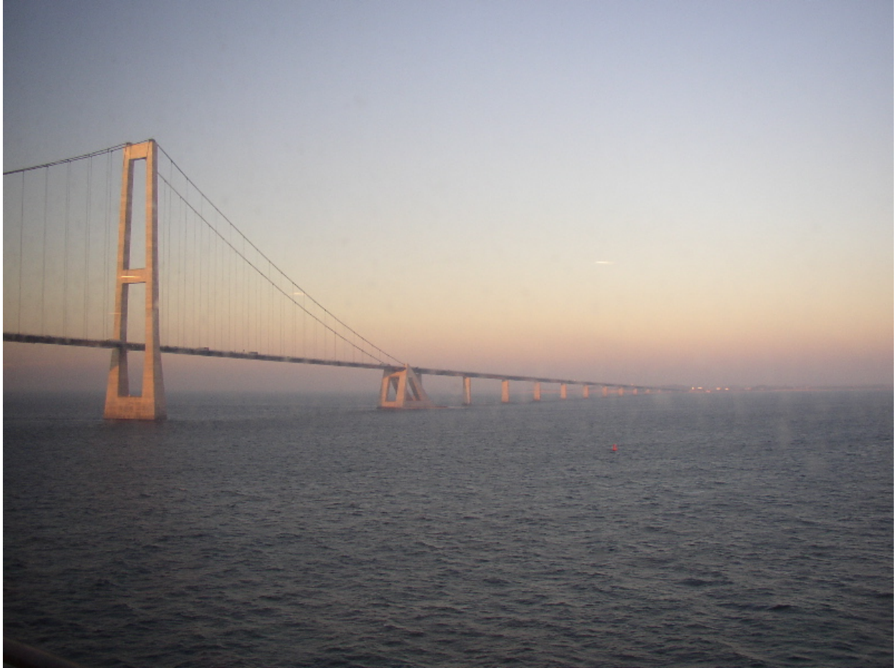
A bridge in Denmark
